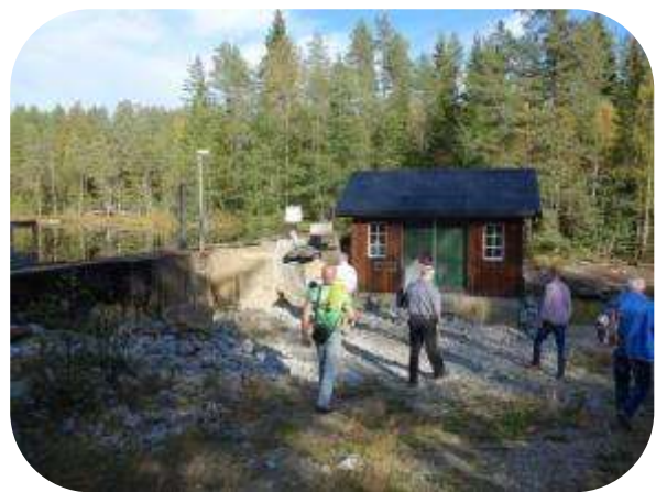
Picture 36: Hydro power plant
