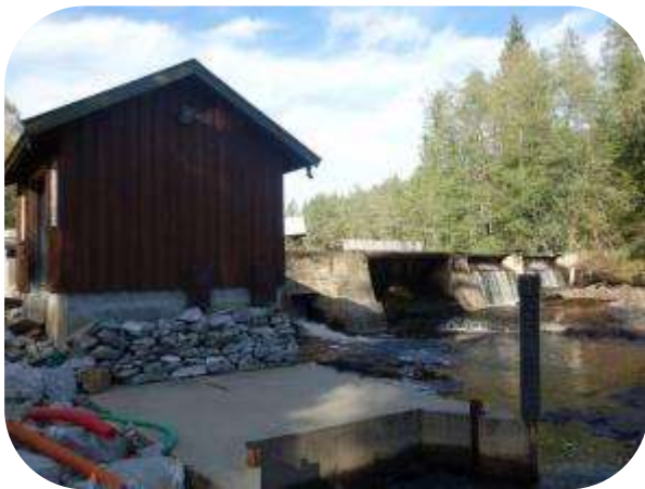
Picture 35: Hydro power plant
