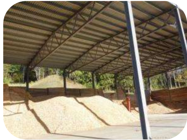
Picture 13: Fuel storage
