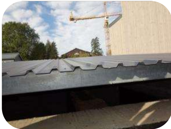
Picture 19: Fuel storage – wood chips
