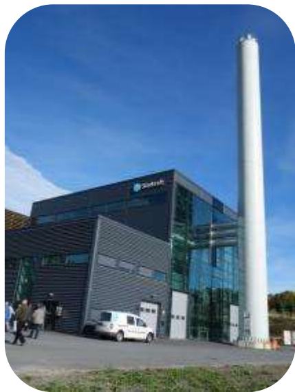
Picture 6: Heating central
