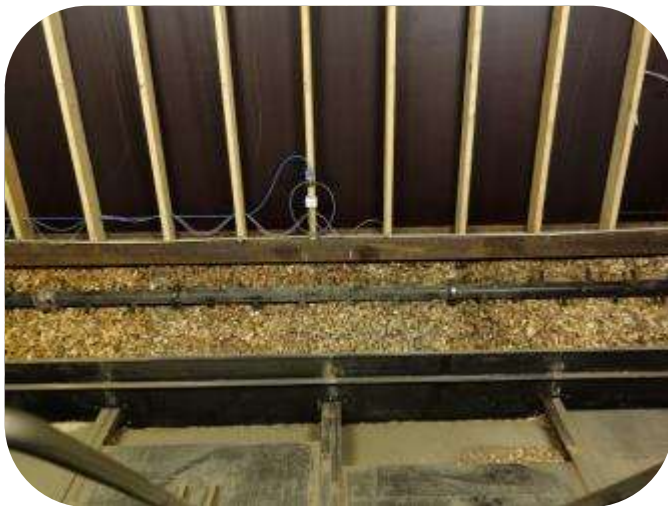
Picture 24: Transport of fuel into the boiler
