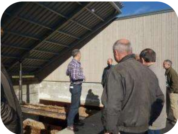
Picture 20: Fuel storage – wood chips
