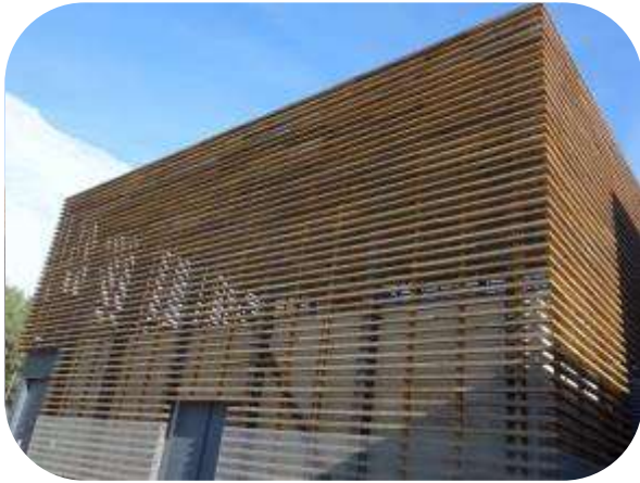
Picture 10: Fuel storage
